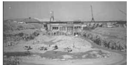
Cowan's Ford Dam Under Development
